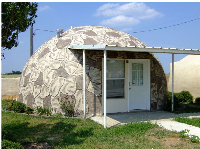
10-24 — Built with an integrated, 3' stemwall, this dome is 24' x 9'. It makes a practical, simply designed, affordable rental unit for one or two persons.
