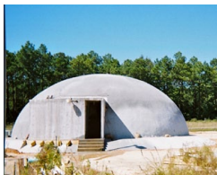
Monolithic Dome at Dupont plant in Delisle, MS. The company's Hurricane Crew of professional damage assessors sheltered in this dome during Hurricane Katrina. The storm did more than $100 million of damage to the plant, but the dome was unscathed. Afterwards, the crew named this dome "The Category 5 Shelter."
