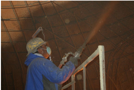
Layers of shotcrete are sprayed over the foam, completely embedding the rebar.
