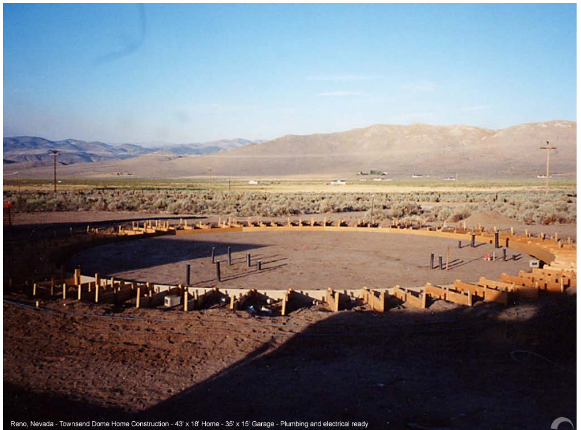
Reno, Nevada - Townsend Dome Home Construction - 43' x 18' Home - 35' x 15' Garage - Forming slab and ring beam
