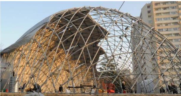
*Figure 2: Créteil gridshell, covering in progress*
