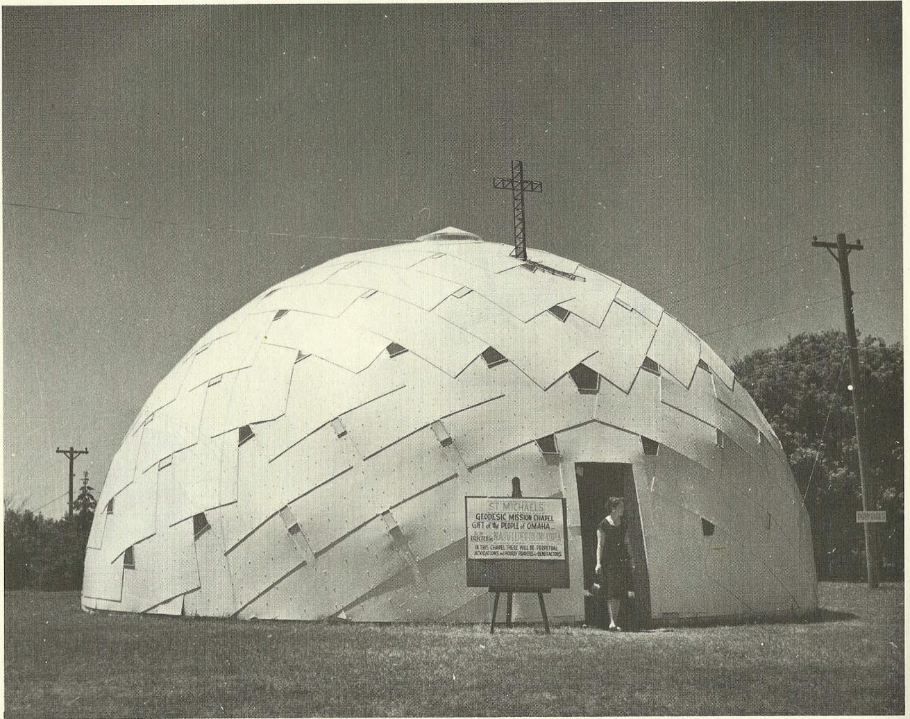
Fig. No. 43 Thirty-nine foot diameter plywood dome. Although not a reticular dome it is interesting to note the use of geodesic geometry and planar sheets of plywood to achieve a dome.
