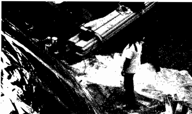
After the slab was completed, this vinyl bag was inflated. With all electrical conduits in position, 6" of 2 lb. foam was applied. A layer of 30 lb. foam was sprayed on the outside. Finally the vinyl bag was pulled down and the inside was painted.
