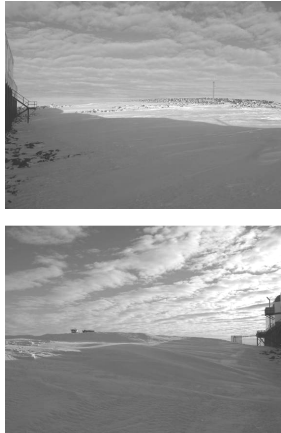
Figure 12: (Top) Negligible snow deposition behind AB link (in line with stair case) with baffles. (Bottom) Extensive snow deposition behind BC link (in line with stair case) without baffles. (Photo: Keith Browne)
