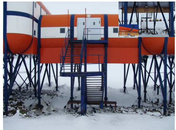
Figure 11: Test wind baffle installation at inter-connecting link (Photo: Stander )
